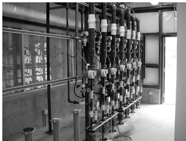
Figure 12. Ground water pumping system – flow meter and conductivity sensor array
